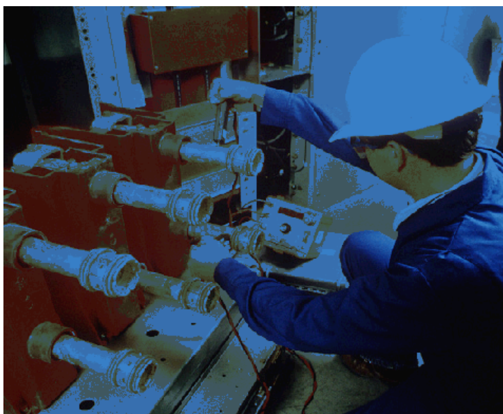
Figure 6-3—Contact resistance testing
