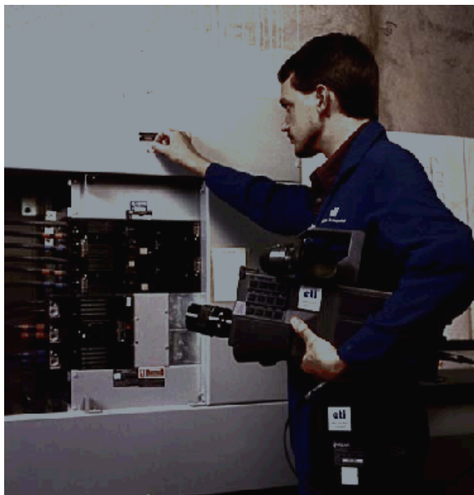
Figure 6-4—Infrared inspection
